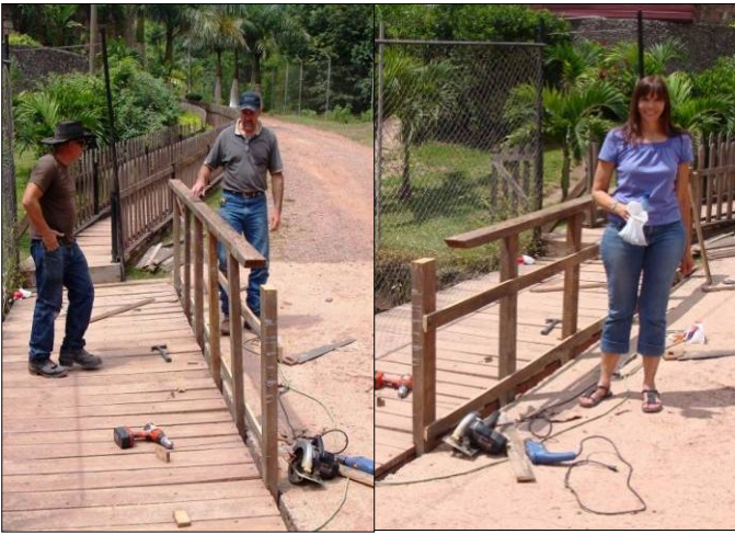
Building the wooden guardrail on our bridge
