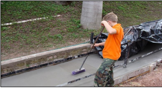
JB helps with the concrete finishing work
